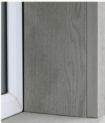
Prefinished Reveal Boards For Window Detailing
