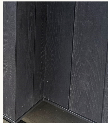
Shadow Line+ External Y Flashing
