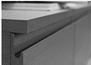
FINGER PULL PROFILE HARDWARE-FREE- J PULL
