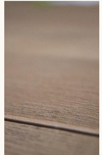
Completed installation with no visible fixing point; the Lastane surface self-heals for a clean finish.
